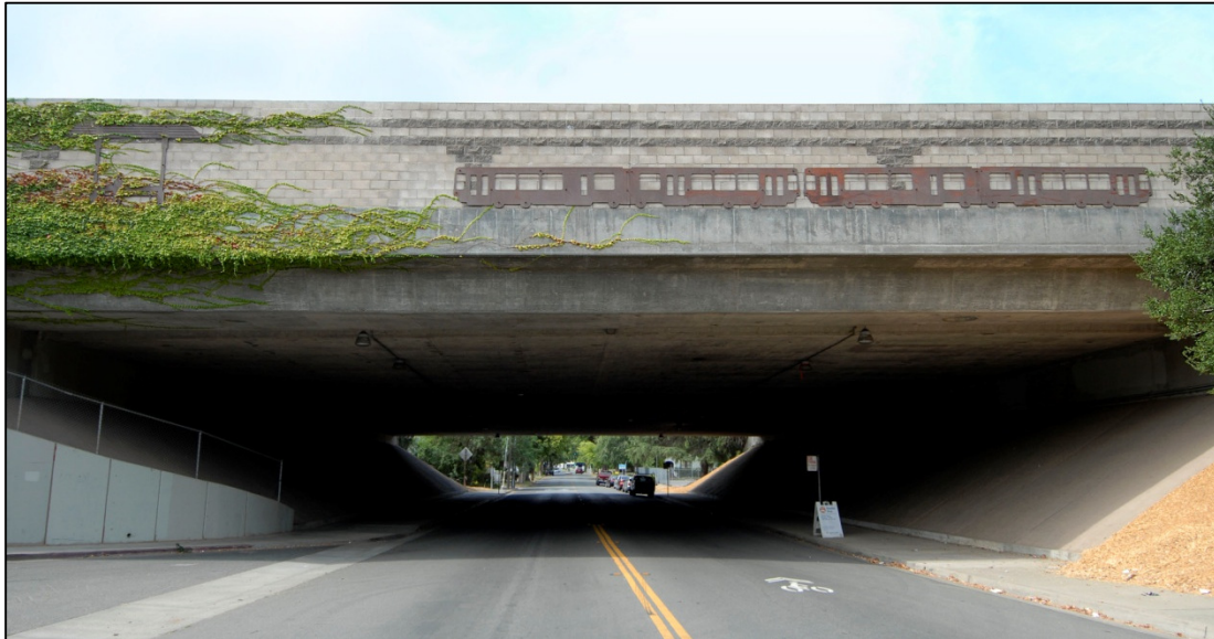
Photo 6 - View from 39 th Street of Existing Sound wall with Metal Art
