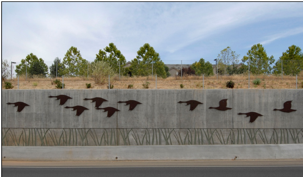
Photo 3 – Retaining with Aesthetic Features
