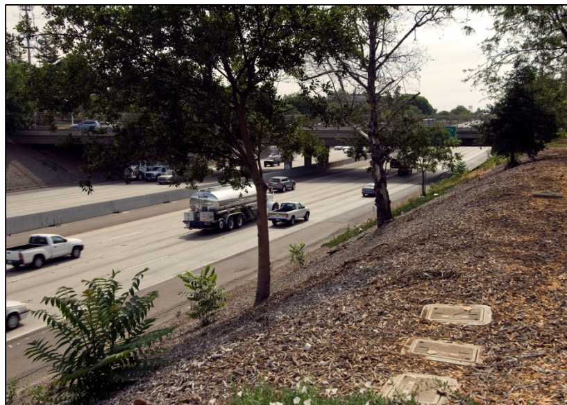
Photo 1 – Depressed Section of US 50 – Showing Steepness of Slope
