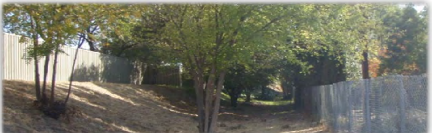
Figure 3 – R/W Conditions A 6 ft metal SW on 8 ft berm exists at the proposed “SW11” and “SW12” alignments. Note that the gap between Caltrans the access control fence is candidate for relinquishment, landscaping opportunity, or other public benefit such as a dog park.
