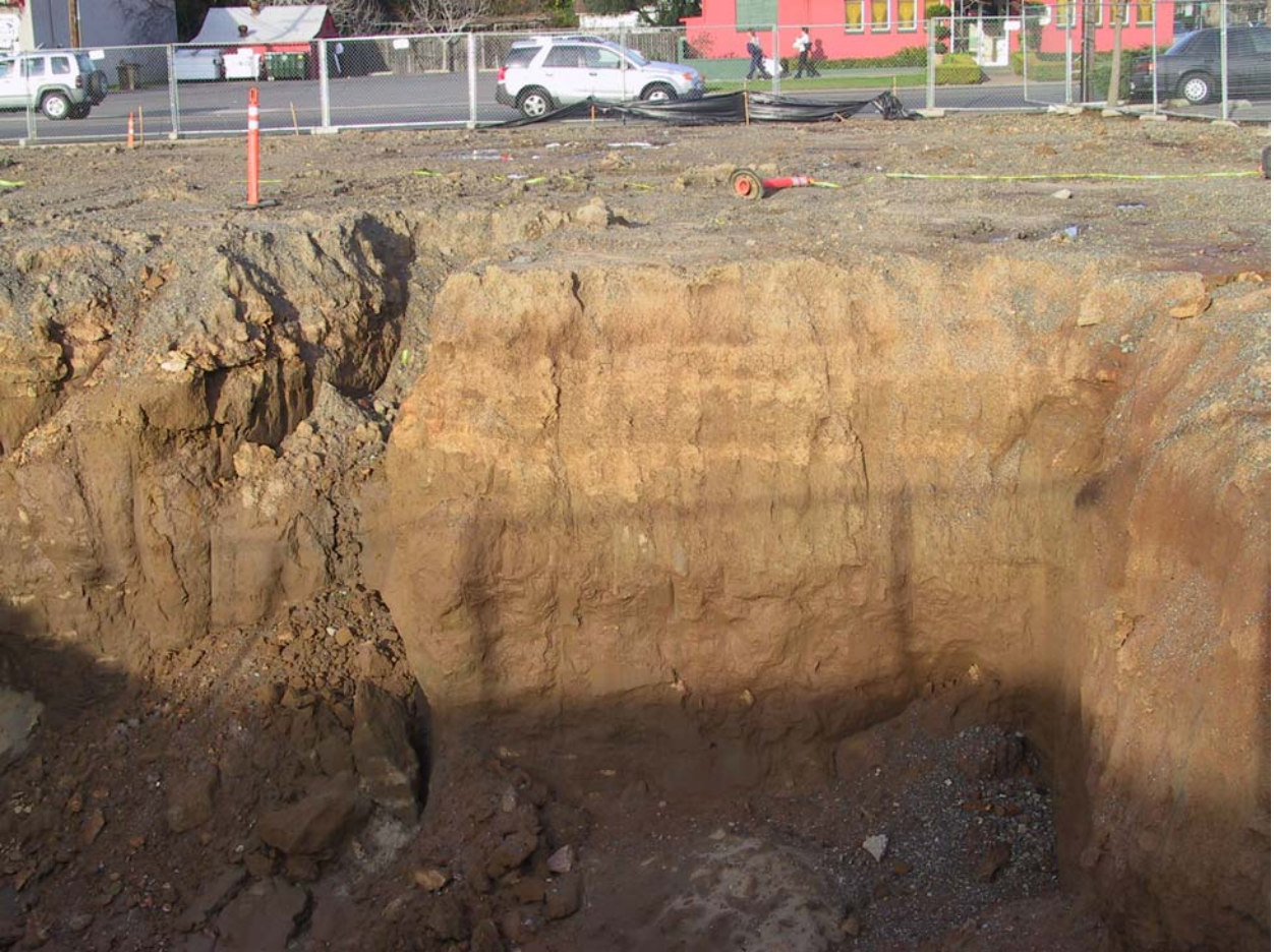
Figure 7. Photograph of Riverbank Formation sediments exposed in a pit for the removal of a leaking underground tank at 5118 Folsom Boulevard, less than 0.40 kilometer (0.25 mile) north of U.S. Highway 50 between 59 th Street and Stockton Boulevard. The light bands in the upper portion of the pit wall are paleosols (fossil soils) containing burrow and root casts and molds (ichnofossils).
